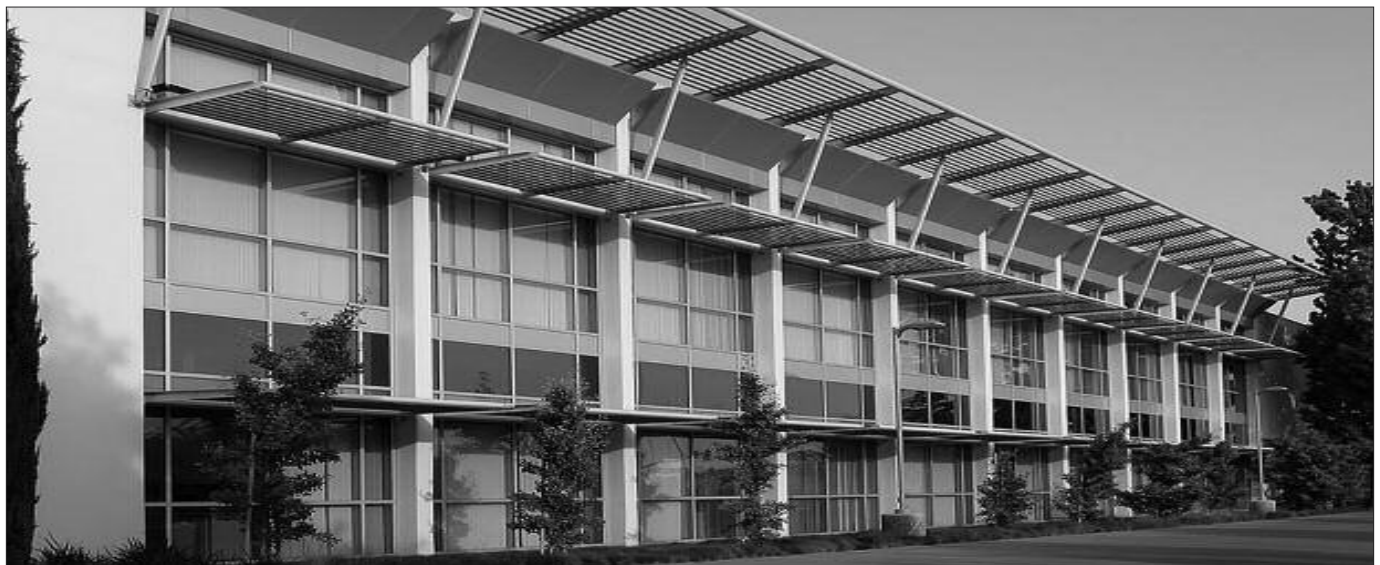
Project: Kaiser Permanente, Downey, CA
